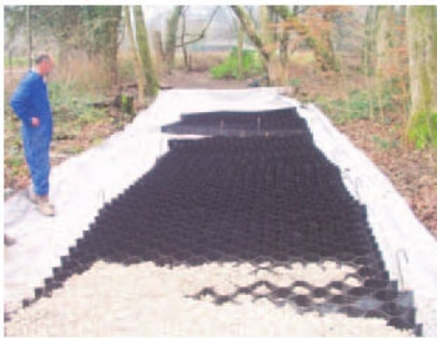
CellWeb during installation.
